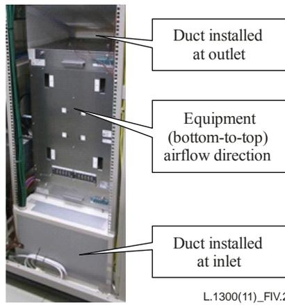
**Figure IV.2 – Example of duct installation in equipment with bottom-to-top airflow direction**
