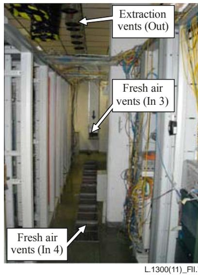
**Figure II.7 – Rack aisle and air distribution system**
